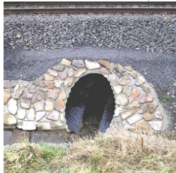
km 234,030 trati Cheb-Hradiště Hel-Cor Trenchcoat DN1000
