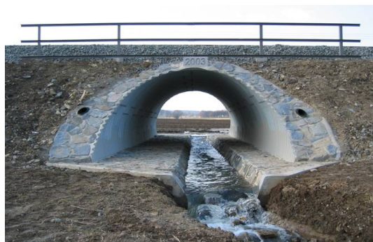
Svitavy Multi-Plate 3,80m x 3,80m
