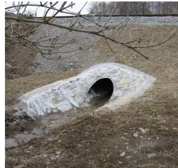
km 34,224 trati Svítavy- Žďárec u Skutče Hel-Cor Trenchcoat DN800
