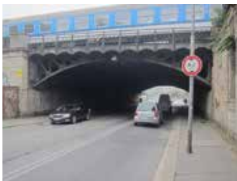
Obr.10 Brno hl.n. most Hybešova
