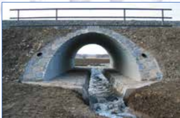
Svitavy Multi – Plate 3,80m x 3,80m
