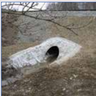
km 34,224 trati Svitavy–Žďárec u Skutče Hel-Cor Trenchcoat DN800
